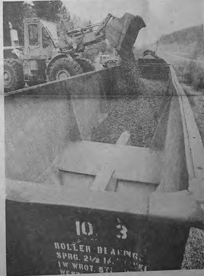
END OF the line for this run is in Campton where four hopper cars are loaded with crushed rock, to be spread along the railbed farther south. About half the line's 72 miles have been repaired.
