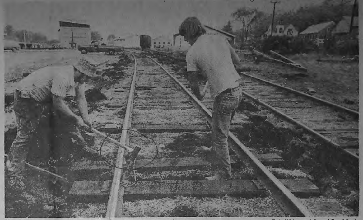
REPLACING ties and adding new bedrock is a crucial factor in attracting the Lakeport maintenance sheds are Dale Whitman, left, and Daryl Lavigne. new business for the Concord-Lincoln rail line. Swinging sledgehammers near
