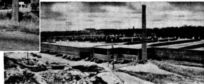
First National Stores Inc. Portland, Me. Food distribution warehouse
