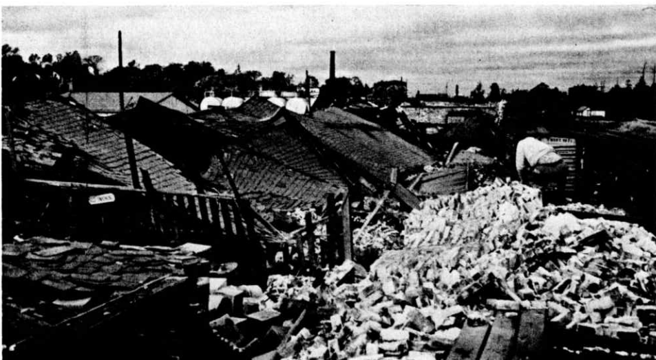
Dover, N. H. Freight House after Hurricane Edna.
