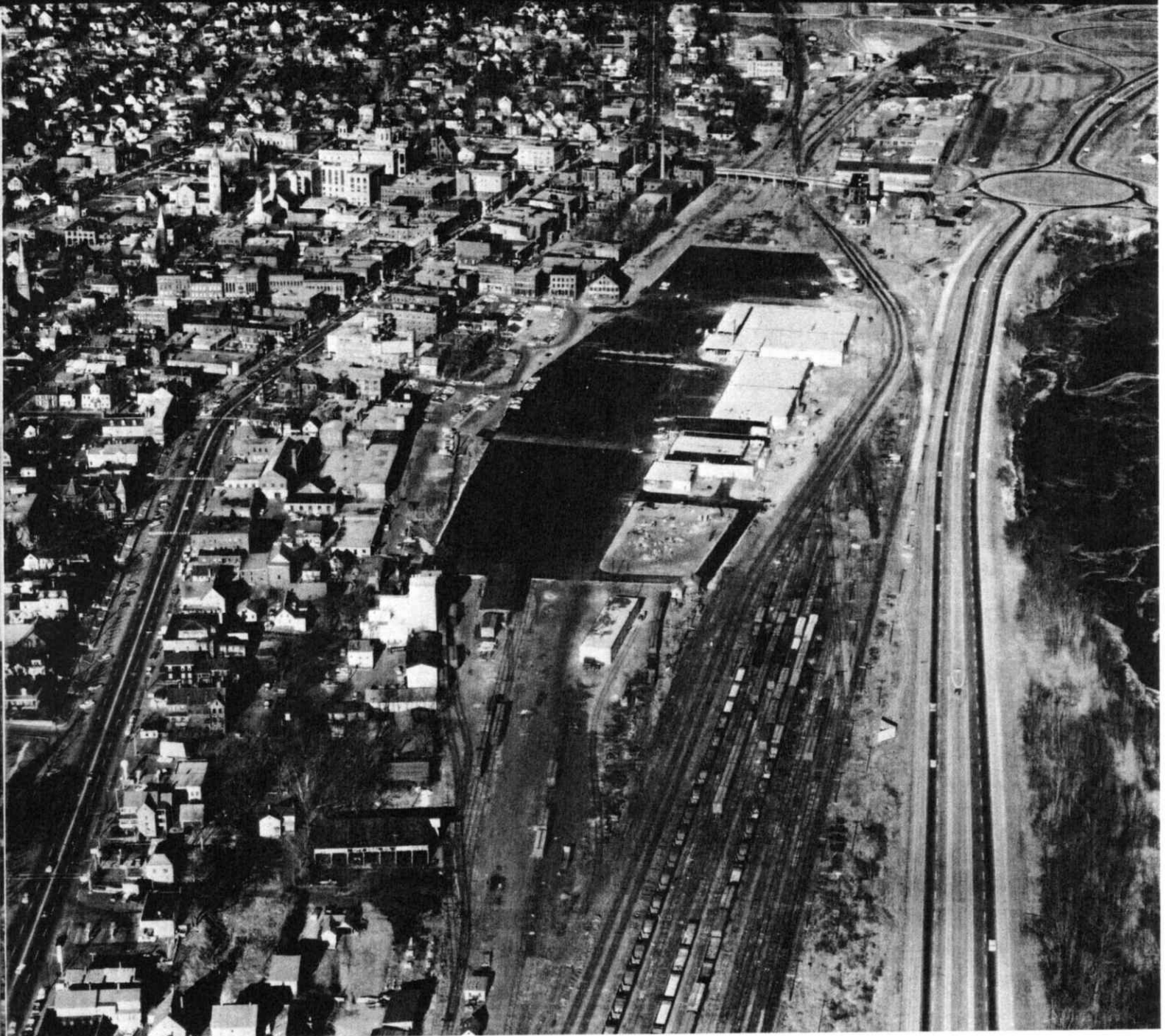
Former passenger station location in Concord, N.H., now a spacious shopping center. Passenger station was located just above center of picture, at point of bulge on left side of black-topped parking area. Streamlined new station is close to top right corner of parking area. Large white building just left of bend in railroad track is new J. J. Newberry Co. store, largest in a rapidly developing complex of department, food and variety stores
