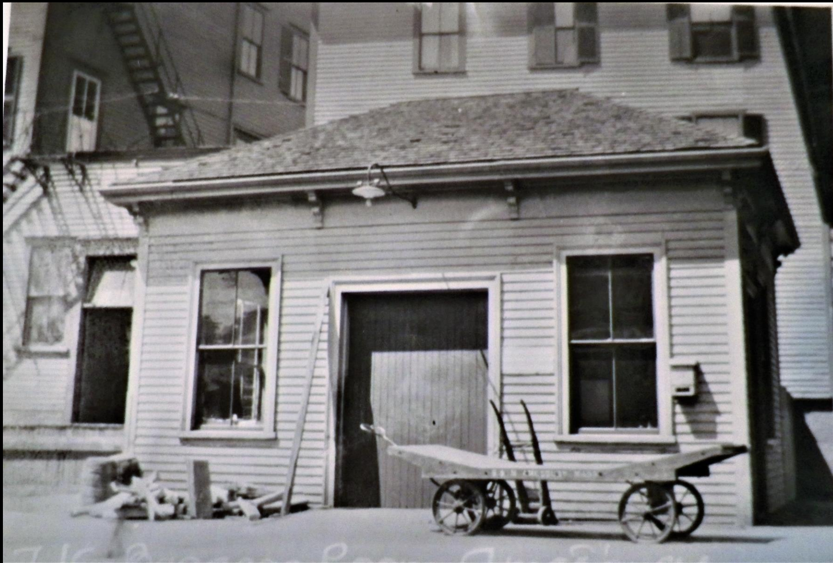
B. & M.R.R. Baggage Shed – Water St, Amesbury 1914
