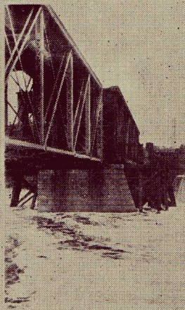
NEW SPAN GOING IN
