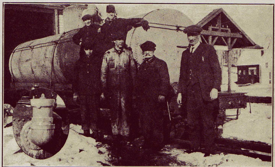
Narrow Gauge Tank Car with Safety Valve Applied
