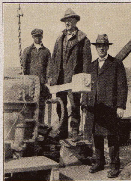
Near the Sand Hogs' Hole—Robert B. Alsop, Superintendent, Foundation Company, who are Building the Piers, and L. E. Thebeau, M. C. General Agent at Bath.
