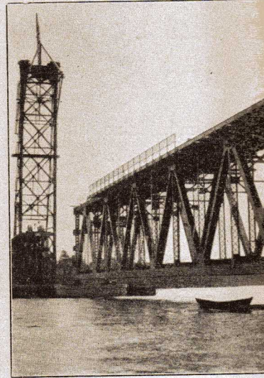
Present Stage of Bridge Construction
