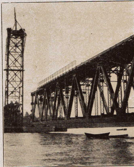
Present Stage of Bridge Construction
