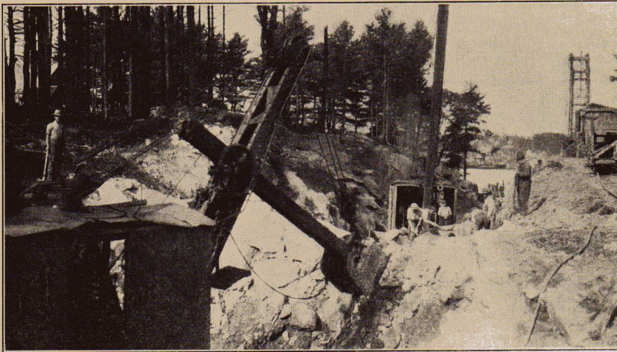
Steam Shovel at Work in Woolwich Railroad Cut
