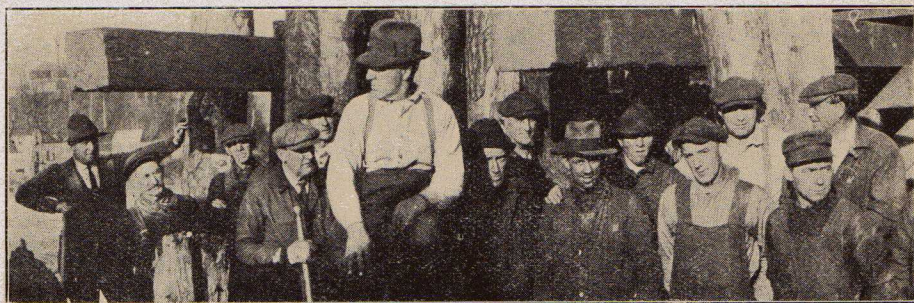
Some of the Crew that Rushed Temporary Bridge to Completion
