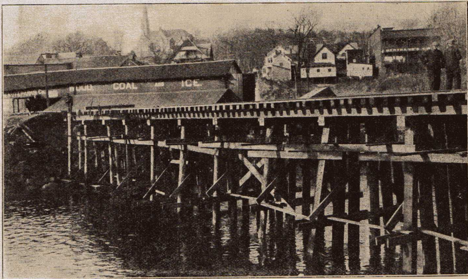
Temporary Bridge over the Passumpsic during Construction
