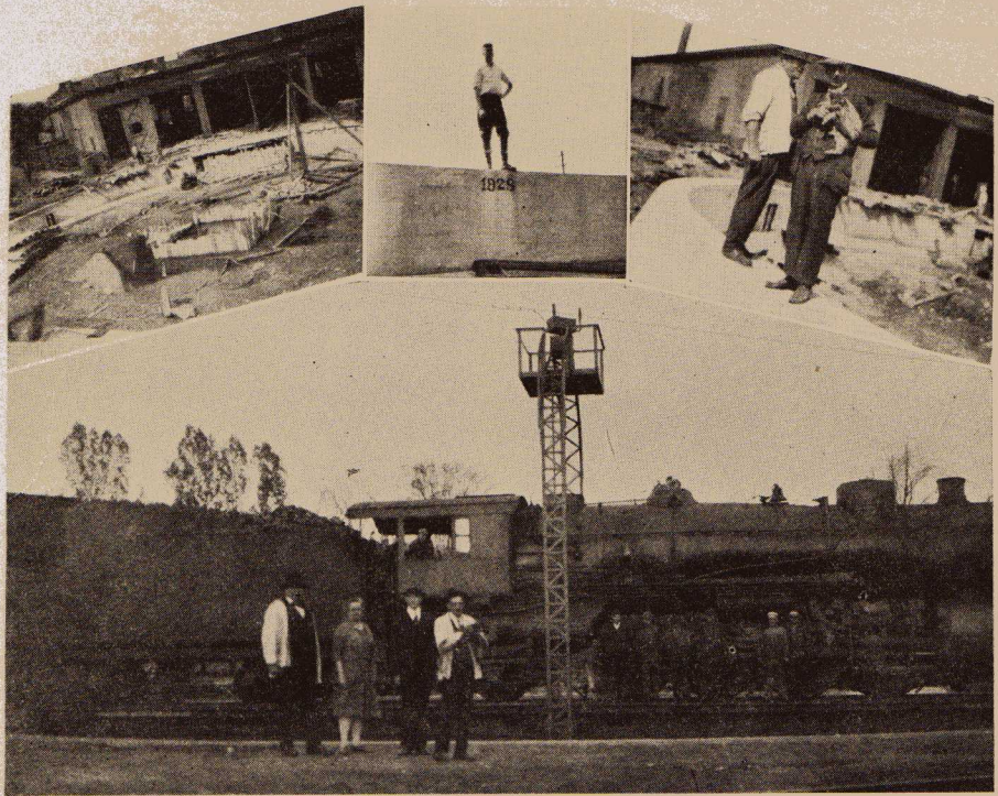
Left upper picture: Foundation of new turntable at Lancaster Round House as it looked September 19.
