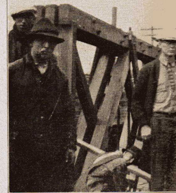
Upper—New span over M Lower—At work on Moose
