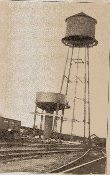
Water Tank at Waterville Yard
