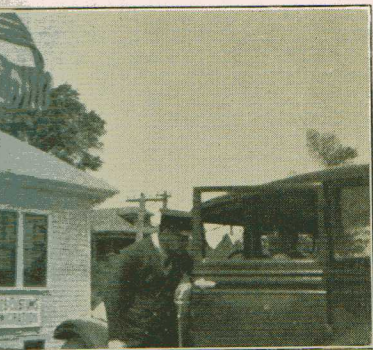
Inspector Bonneau on the Job
