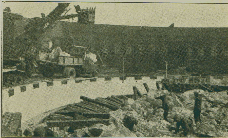
Just after the temporary circle was "blasted out"
