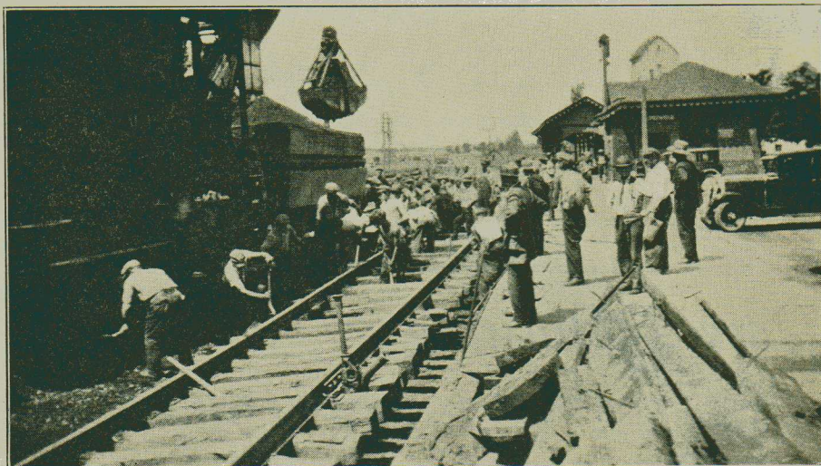
Lowering main track at Pittsfield
