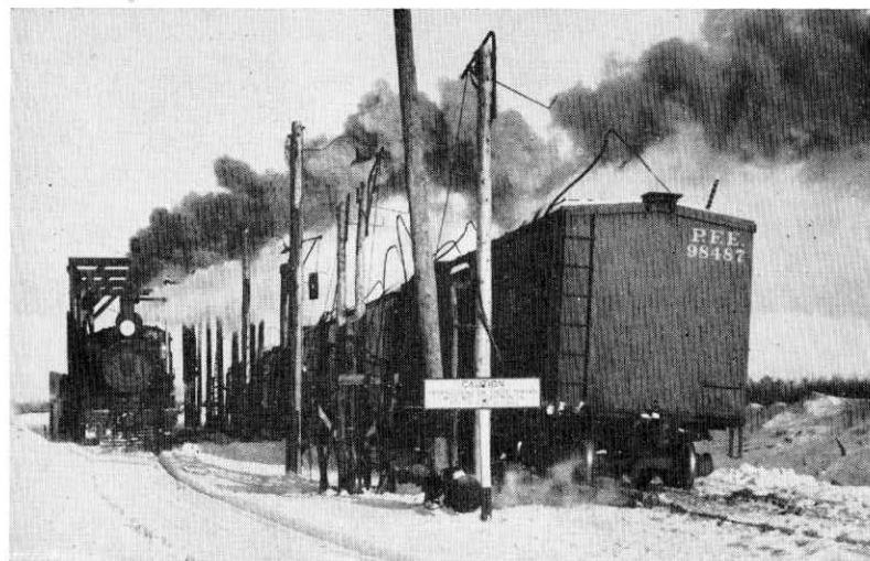
De-icing "reefer" cars at Northern Maine Junction. Steam generated by the standing locomotive is forced through pipes and hose into five cars at a time, melting the ice from bunkers so they can be used for potato shipments.
