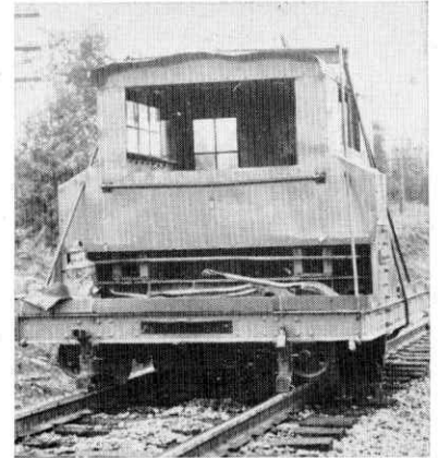
Ballasting machine operated by one man which moves along track one tie at a time and drives ballast down between and under ties.
