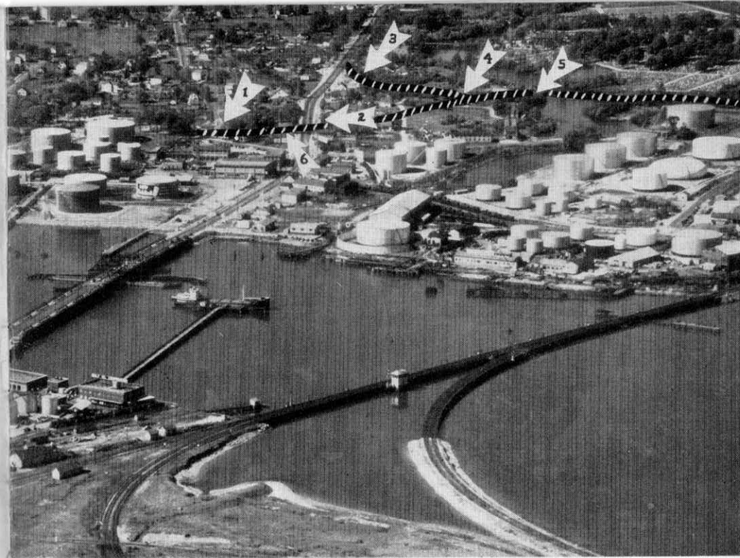
THIS GANNETT AIR PHOTO shows the Vaughan Bridge and Railroad trestle as they exist today. Arrows indicate buildings that will be moved for the highway approaches. Our wye at right bottom will be taken up
