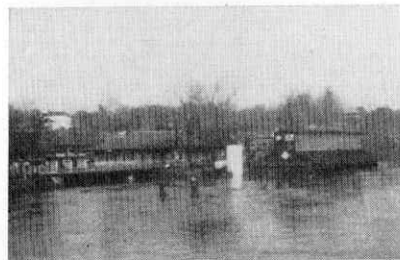
SURROUNDED by water during the 1953 Spring floods was the Gardiner passenger station
