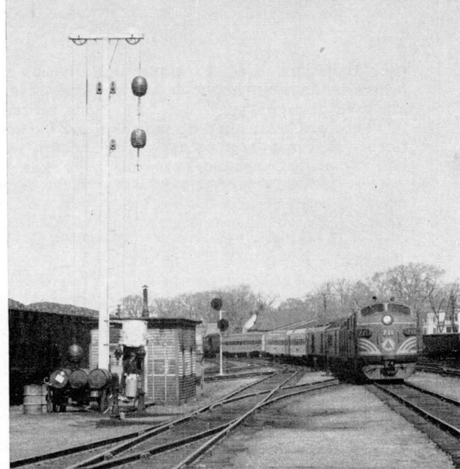
Receiving a proper indication on the ball signal east of Portland Union Station, Train No. 14 from Bangor proceeds to enter the station.
