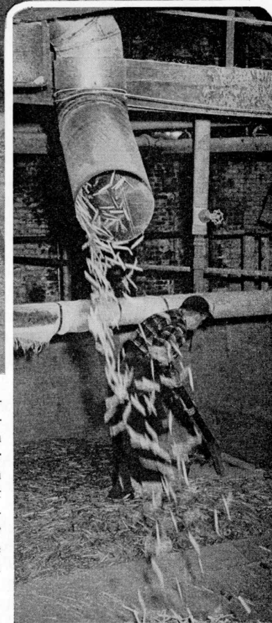
THE OPERATION AT THOMPSON'S POINT—The Forster Manufacturing Company-Maine Central clothespin "pipeline" ends at Thompson's Point after the pin woods have been hauled from Mattawamkeag in the MeC's new covered hopper cars. At left, Maine Central draftsman Laurence Sparrow, in raincoat, watches as preparations are made to unload the first car. The electrically-driven blower is housed in the small trackside building. Above, the pin woods are blown from the car up this pipe to the roof of the assembly plant and then cascade into bins as shown at right. The pin woods then flow through more pipes to the assembly machines on the floor below.
