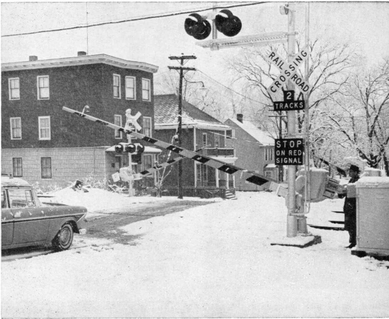
NEWEST GATES —Automatic highway crossing protection went into service early in March on Coyle street in Portland, the first of three residential streets where automatic gates will replace manual systems in the near future. J. F. Stanford, signal engineer, demonstrates the new gates.
