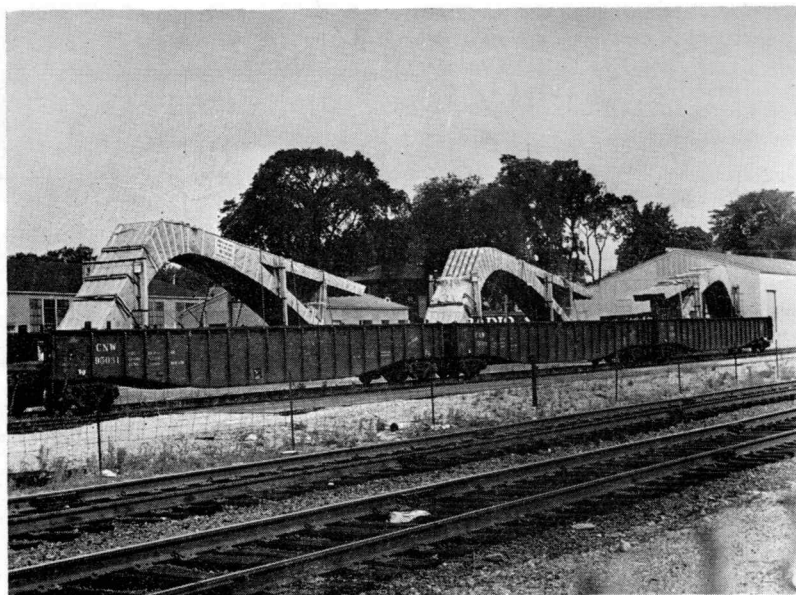
ARCHES FOR ST. PATRICK'S —Portland Terminal Company crews spotted these cars loaded with carefully-wrapped wooden laminated arches in early July. They'll be used in construction of the new St. Patrick's church on outer Congress street in Portland.
