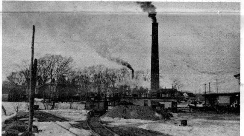
PORTLAND SCENE . . . 1914 —Bill Grace, PTCO. plumbing shop, supplied this old picture of the area now occupied by the maintenance of way and electrical shops behind the former Union Station area. Congress street is in the distance, and the old heating plant stack rises near the center. Bill asks if anyone can tell him what the other stack is . . . the one in the far background.
