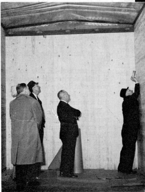
Looking for leaks
