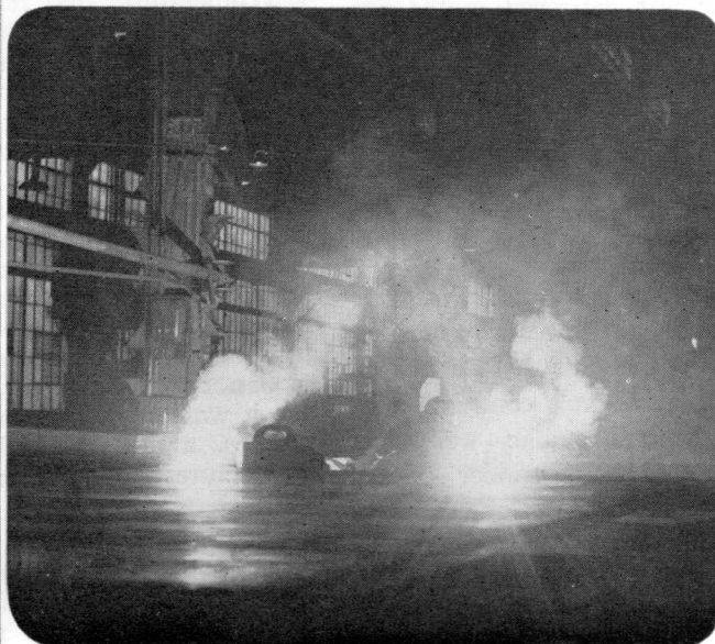
Welders work on car side
