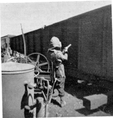
NEW USE FOR OLD TURNTABLE— Not a man from Mars but Painter Helper Don (Red) McCaslin in an air conditioned hood, grit-blasting a section of a turntable, taken from the Lewiston engine house, preparatory to being painted and installed on the Eastern Division as a bridge section.
