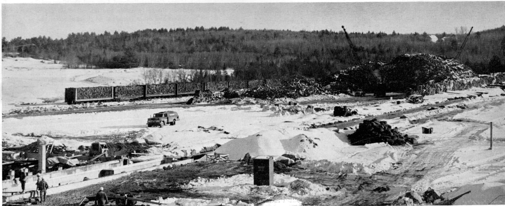
JAY PULP PILE GROWING—Pulpwood is being stockpiled rapidly at the site of the new International Paper Company mill at Jay, much of it arriving in the new, 72-foot "Paul Bunyan" bulkhead cars now in service on the MeC and BAR. As of January 6, a total of 267 carloads—roughly 6,000 cords—had been delivered to the new mill site, where production is scheduled to start in the fall. This picture shows the wood yard area, with several carloads awaiting the attention of the IP unloading crews.
