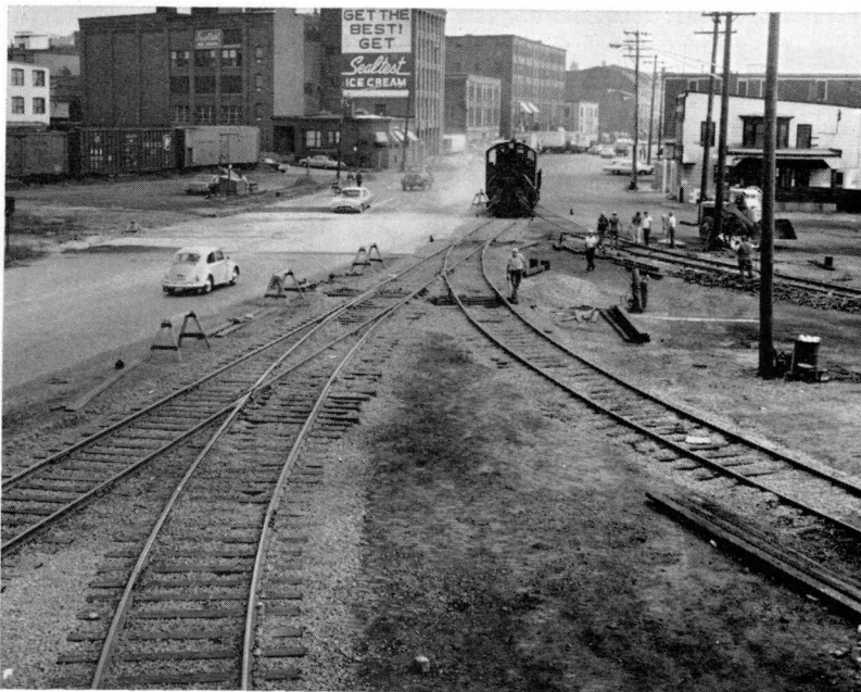
WATERFRONT IMPROVEMENT —The part of the Portland Terminal Company in continuing efforts to upgrade Portland's waterfront has been the raising of track to accommodate a new surface for Commercial street, begun last summer. The job is nearly completed.
