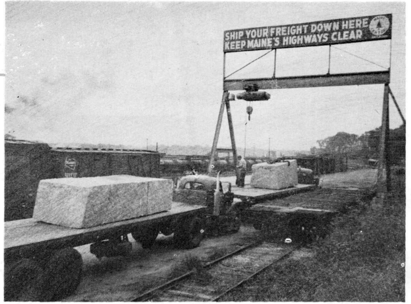
BOUND FOR OHIO —Stone from the Deer Isle Granite Corp., Stonington, was loaded aboard a flatcar last month bound for Ohio, where it will be used in a mausoleum. Each of these blocks weighed about 17 tons, and were loaded with the overhead crane in the Bangor freight yards.
