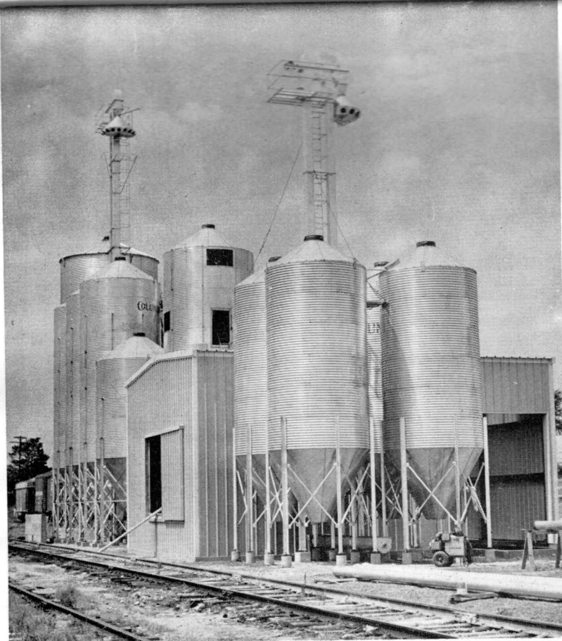
NEW ROCKLAND PLANT —These gleaming tanks and buildings have risen near the Maine Central engine house at Rockland, and will soon be turning out mixed feeds for the H. K. Webster Company and the poultry and dairy farmers of coastal Maine. Whole grains will be delivered by rail, and bulk trucks will handle the products.
