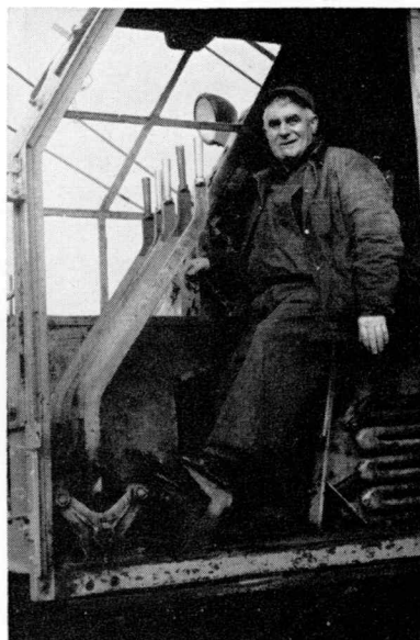
A busy little man with a big job is Rocco Risbara, Crane Operator in Maintenance of Way Department, Waterville.
