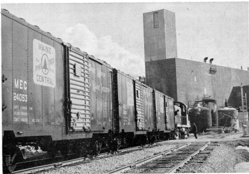
FOR FINISHED PRODUCTS —These Maine Central box cars, designed for woodpulp shipments, are being placed by the switching crew for loading at the expanded mills of the Penobscot Corporation at Great Works. One of the new buildings is shown in the background.
