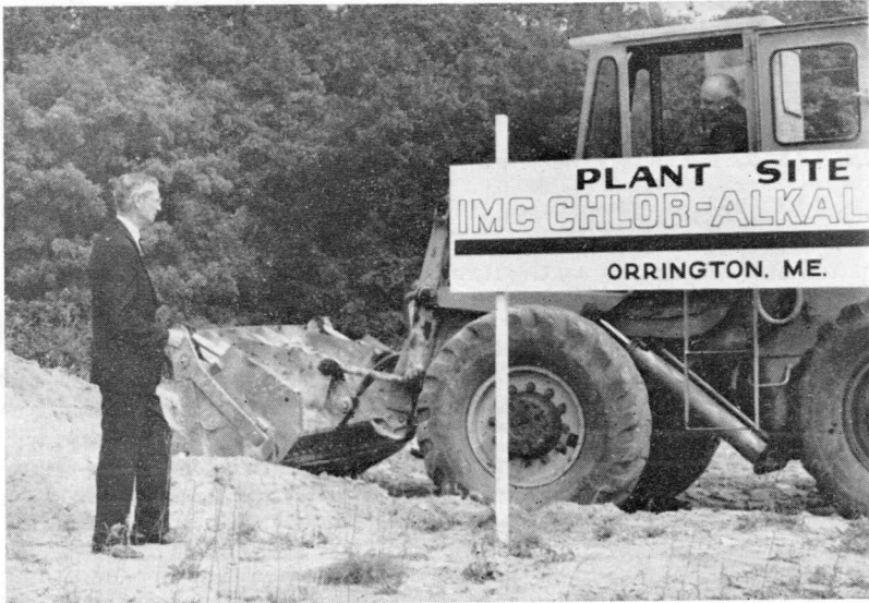
BREAK GROUND AT ORRINGTON —Bland B. Button, Jr., president of IMC Chlor-Alkali, Inc., directs Morris McDonald, first selectman of Orrington as the latter moves the first earth at Orrington to signal the start of the firm's new $9.5 million plant.
