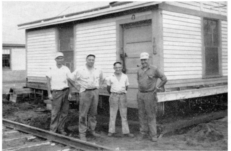
UP IN THE AIR —Brunswick Car Shop is shown all up in the air over the new sills and floor being put in by Pomeroy's Crew. Left to right, R. B. Ridgell, Morris Fish, L. R. Bernier and Dana Pomeroy.
