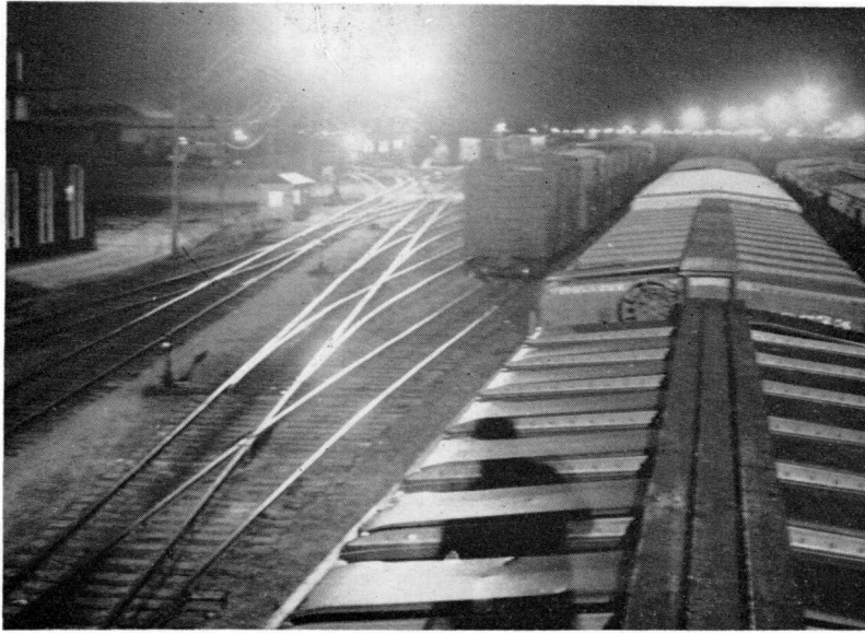
THE YARD AT NIGHT —Brightly illuminated by the new lighting system, Waterville Yard presents this view at night, looking west toward the city from the Shops area.
