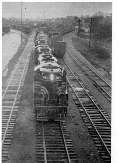
EAST YARD, WATERVILLE —Birds-eye view from Signal Tower on Allen Street, east yard, Waterville, of B-11 setting off cars.
