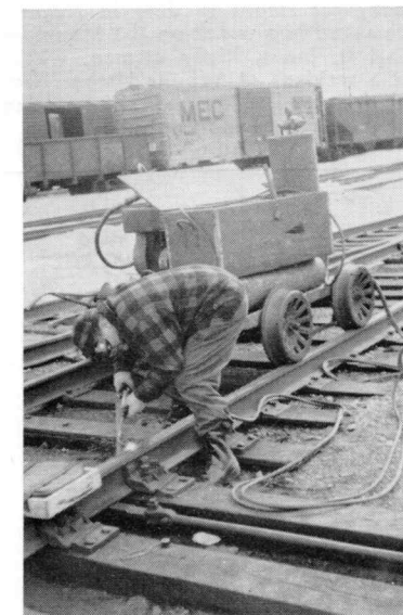
MAN FROM MARS —Chester Haskell welding switch points at Waterville Yard.
