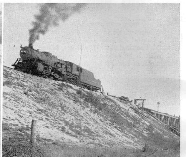
Locomotives were used at one point in the operation to raise and hold the bridge.
