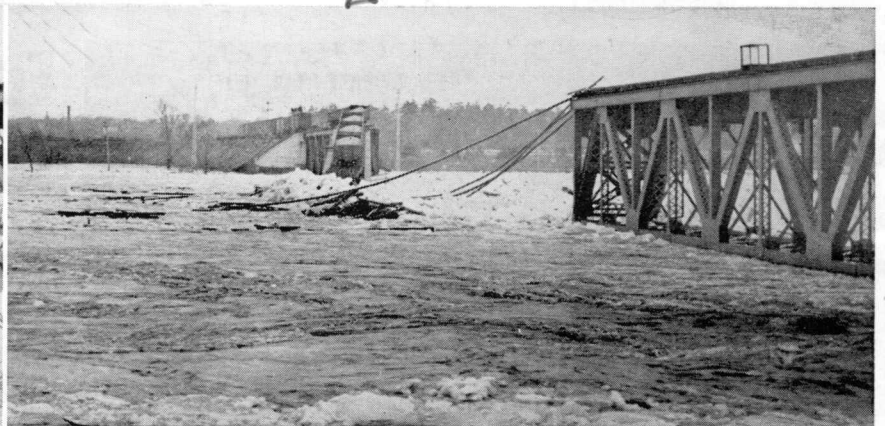
One section at a time, the long span toppled into the river and sank, some of it nearly 100 feet downstream from the piers.
