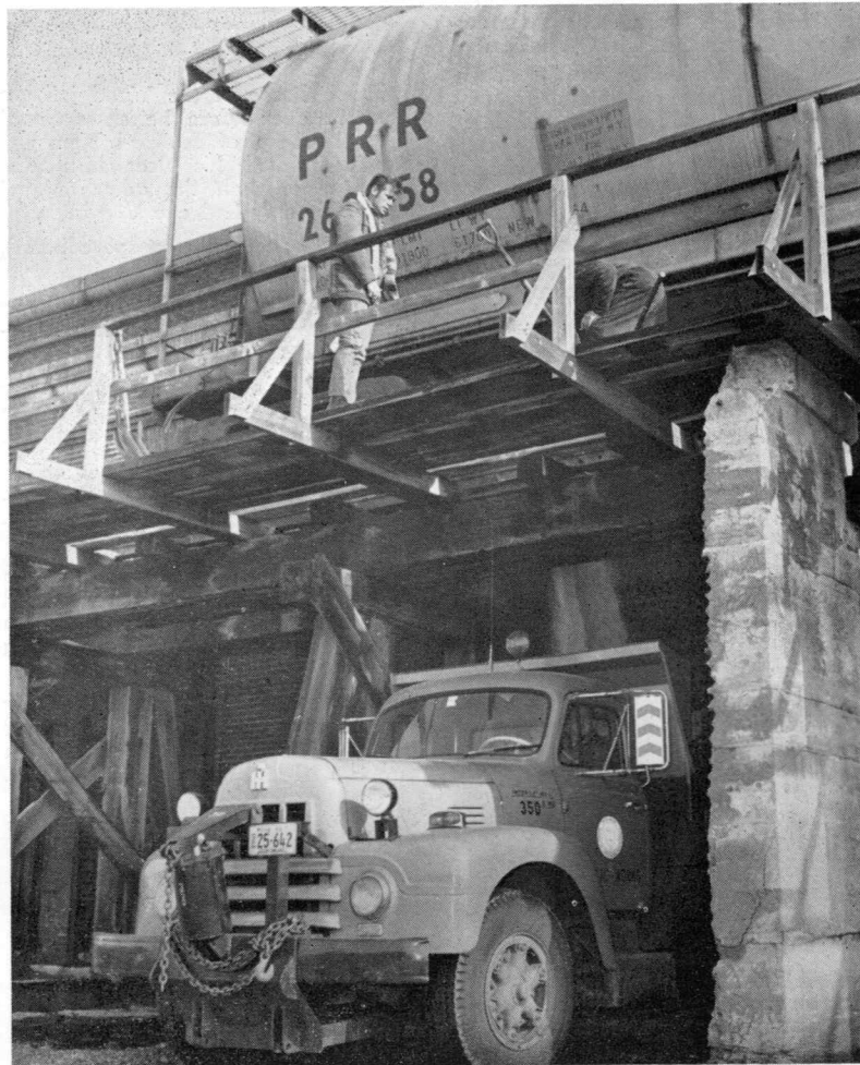
SALT FOR THE CITY —A City of Portland Public Works Department truck loads salt at the W. H. Shurtleff Co. storage facility that for many years served as the heating plant for Union Station. The salt is part of the thousands of tons used annually in Maine for ice control.
