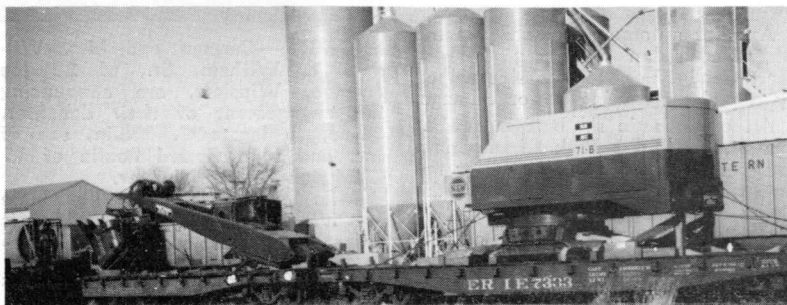
AT WORK IN THOMASTON —Arriving at Rockland recently was this huge new Bucyrus Erie power excavator 71-B, later assembled at the Dragon Cement plant in Thomaston. The machine is now working at Dragon's new plant site, its 4½ yard bucket speeding up production.
