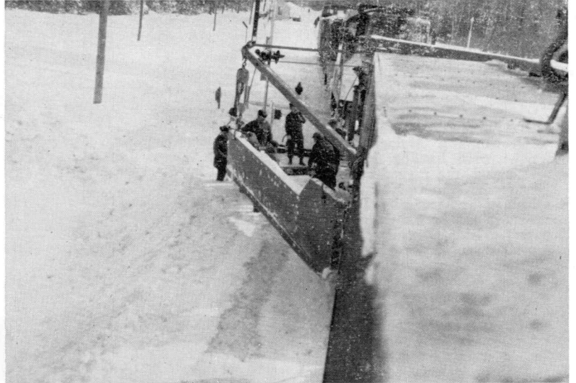
AT FOREST —Preparing to move west to spread the snow off the north passing track.
