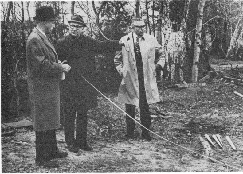
EARLY START ON NEW SHREDDER PLANT —Not long after the winter's snow disappeared, officers of National Metal Converters, Inc., visited the site of their proposed metal shredding plant at Leeds to plan location of buildings and other facilities. From left, Charles C. Rivers, MeC industrial development manager; Irving Zaitlin, vice president, and Harry Zaitlin, president of the new company.
