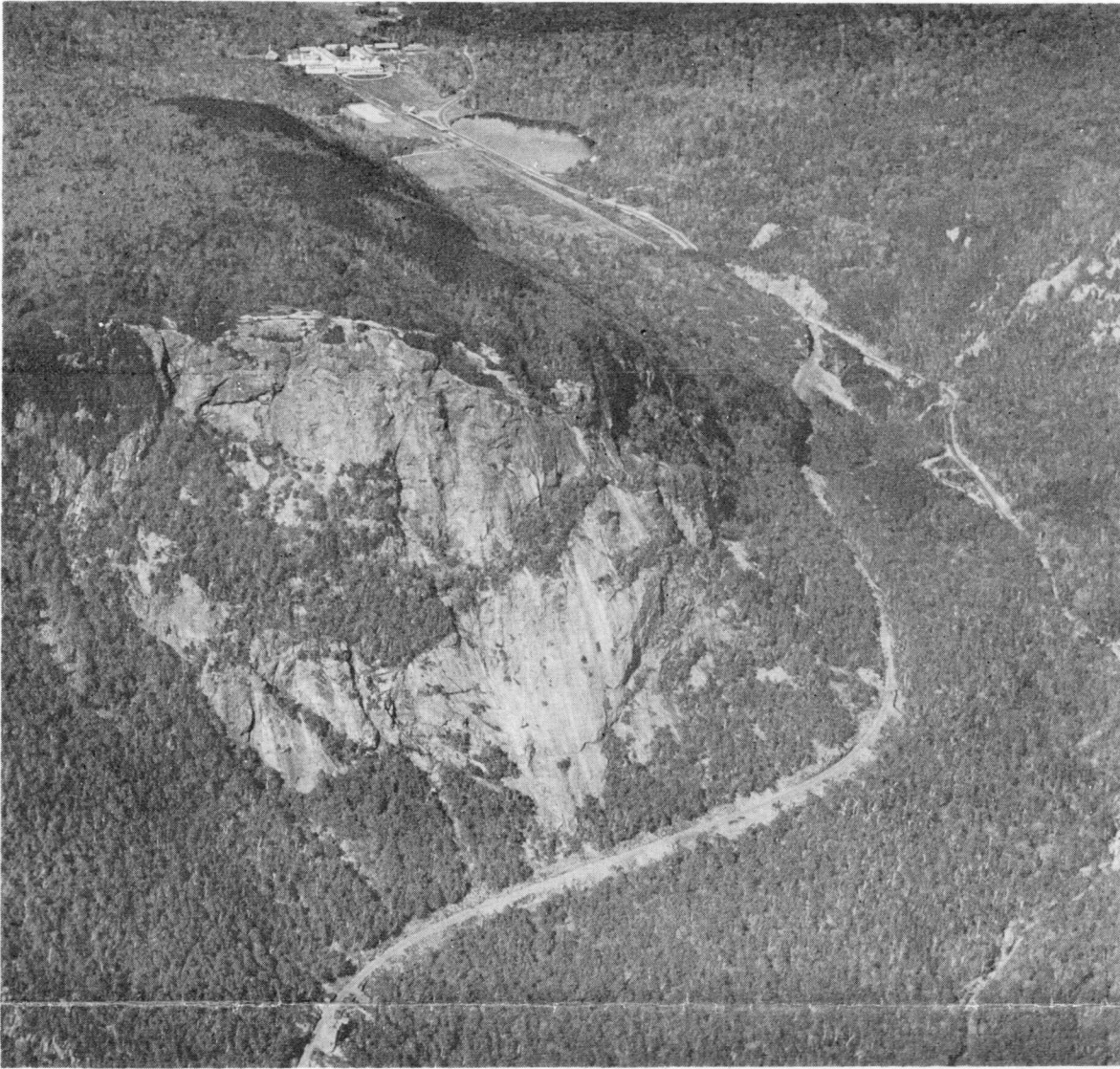
The Crawford House, upper left, is dwarfed in this air view of Crawford Notch area, showing Mt. Willard at the center with MCRR tracks curving around its side and the famous trackman's house perched on the mountainside in the foreground. Route 302 runs along to the right, parallel to the tracks.
