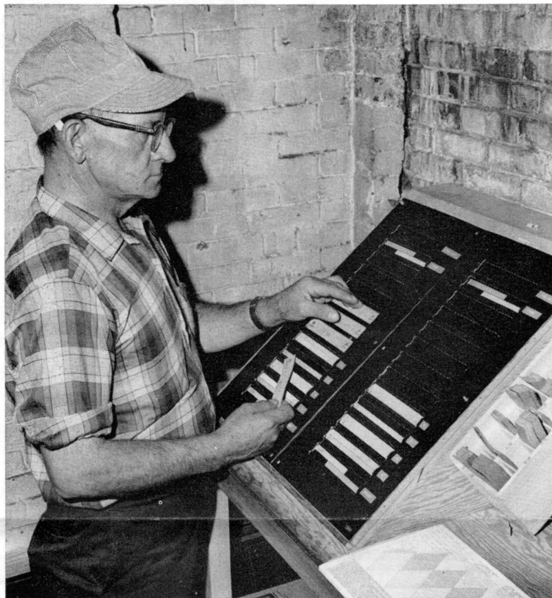
"SERVICE STRIPES"—Warren Johnson, Waterville Shop applies car numbers to a pair of black aluminum plates as part of the ACI system project. Maine Central's AAR "reporting marks" are the figures 0456 and the Portland Terminal Company's, 0619. At lower right in the foreground, is a Quik Trak Validity Digit Calculator Sheet designed to make the job simple. Projection on a graph-like chart produces a figure total designed for error-free can identification.
