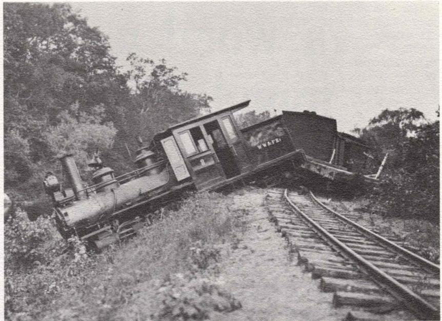
Operations on the Wiscasset, Waterville & Farmington were abandoned on June 15, 1933, when the early morning train derailed near Whitefield. Seven years later, after the rails had been torn up, No. 8 still rested in this same location.
