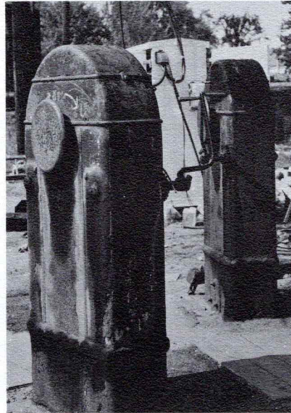
Old Style hand cranks used to operate manual gates.
