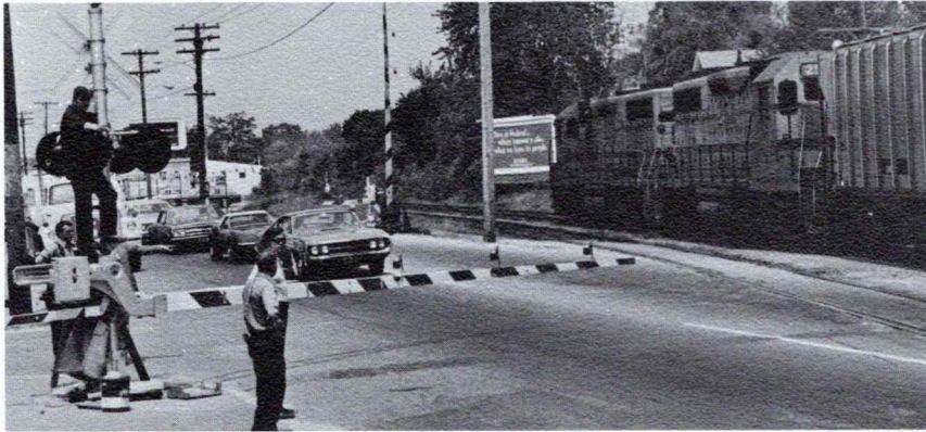
The first train through the new automatic crossing gates at Woodford's Corner in Portland. Maine Central signal department employees carefully monitor the first operation.
