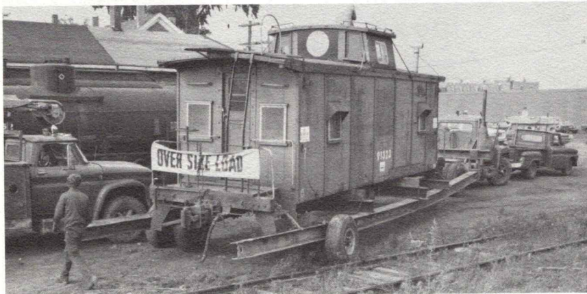
The Caboose, which has been picked up and lowered onto mobile "I" beams, begins its 5-mile final leg over the highway moving by Rockland City Hall, (former Maine Central passenger station).
