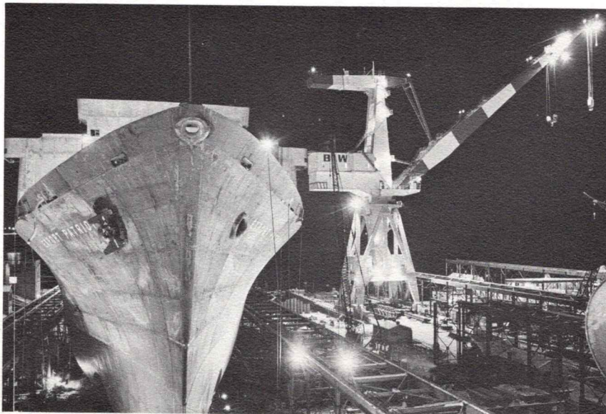
The third in a series of three 610-foot containerships has been launched by Bath Iron Works. In the background is the new BIW 200-ton capacity crane, the largest of its type in the United States. BIW photo by Tom Jones.
