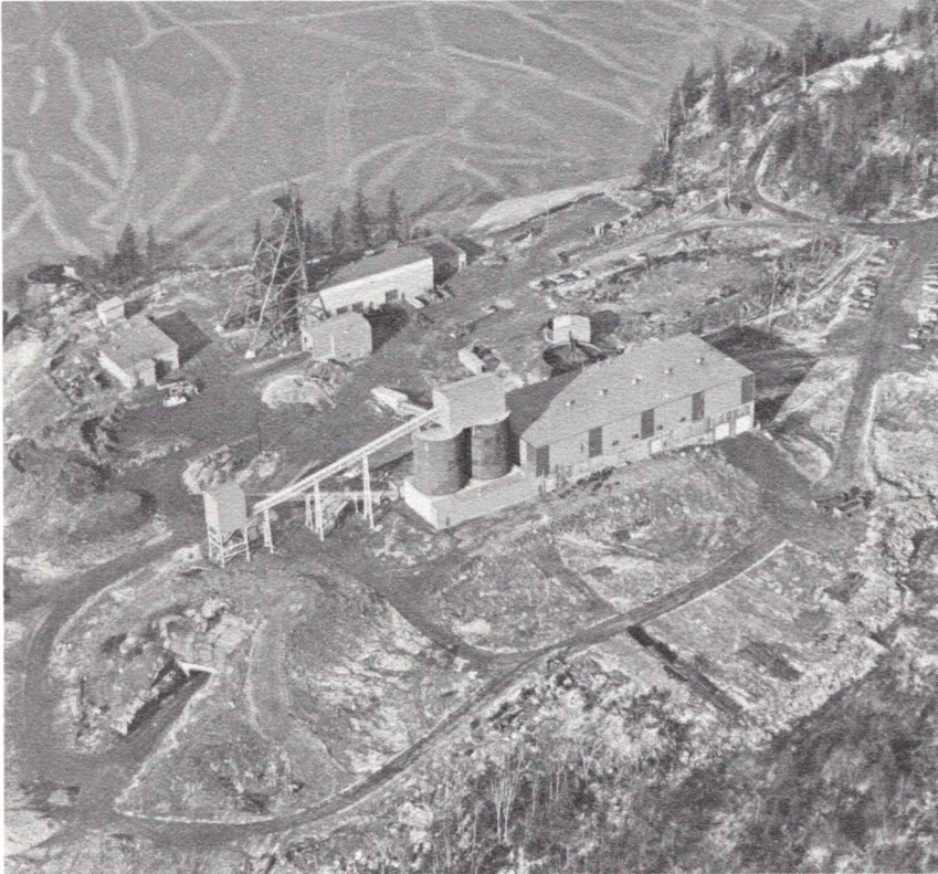
View of the zinc-copper mining operation in Blue Hill. Note the mine entrance in the lower left corner. The buildings in the foreground are for the concentration process. The mine itself is under the pond. (photo by Hugh W. Bowden).
