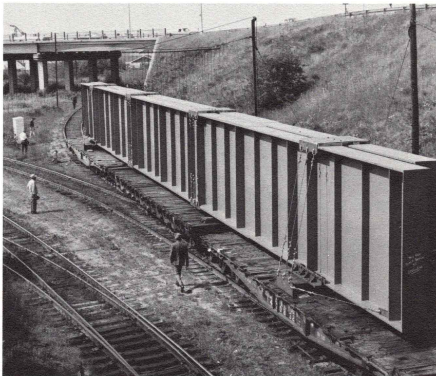
Two steel girders, nearly 140 feet long and fabricated by Bancroft & Martin, Inc., in South Portland, were taken by Maine Central special train to New Hampshire to be used in the construction of a Boston and Maine railroad bridge. The 120-ton load was carried on two six-axle, heavy-duty flatcars with a four-axle flatcar used in the middle to properly space the load.
