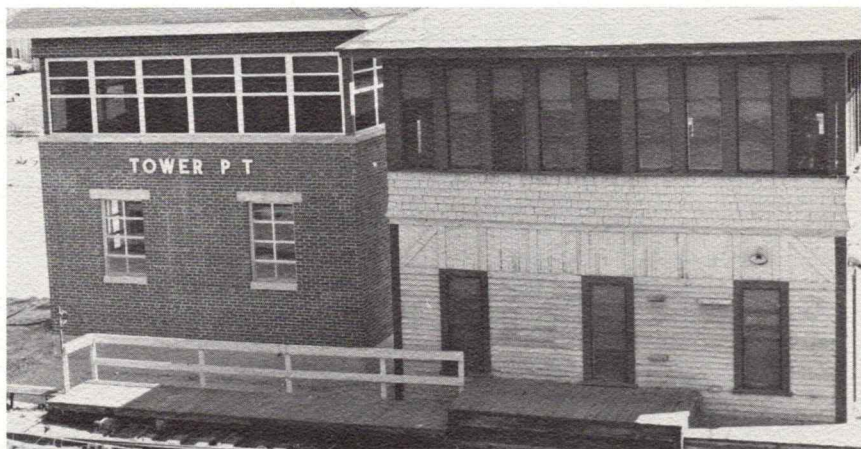
The new, modern Tower PT stands beside old Tower 2 at the east end of Rigby Yard. The new facility, of brick and concrete construction and completely fireproof, replaces three older towers.
