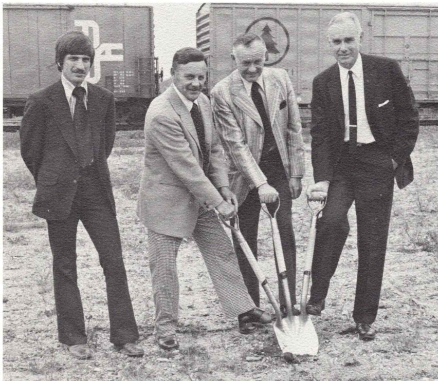
A three-handled shovel breaks ground for the first occupant of the Railroad Industrial Park in Westbrook. Left to right are: Ronald P. Russo, building consultant for the Sheridan Corp., the contractor for the facility; Joseph Morin, president, J. L. Morin Co.; Westbrook Mayor Donald J. Brydon; and E. Spencer Miller, Maine Central president.
