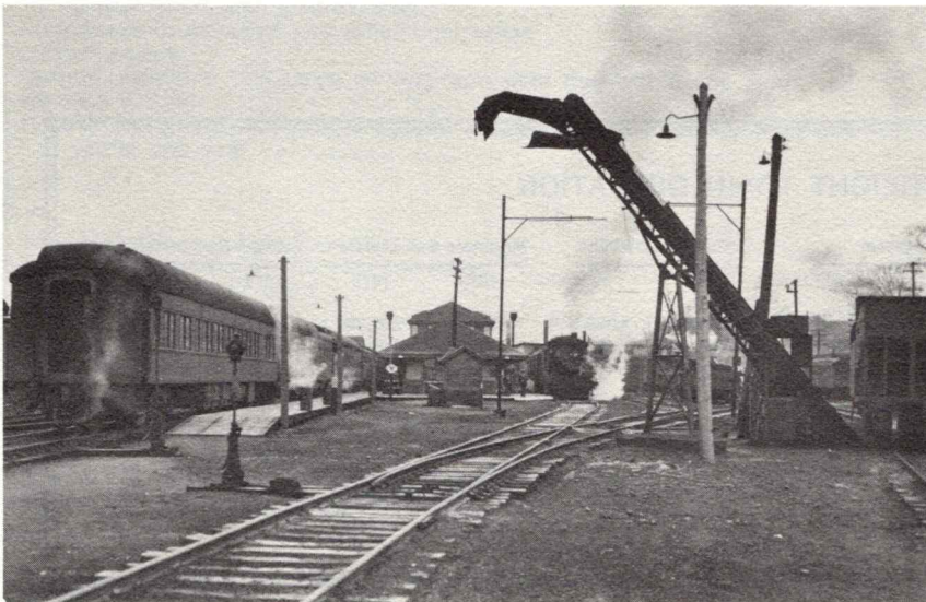
Vanceboro Station as it looked in 1944. Maine Central has reached an agreement to sell its line from Mattawamkeag to Vanceboro to Canadian Pacific.
