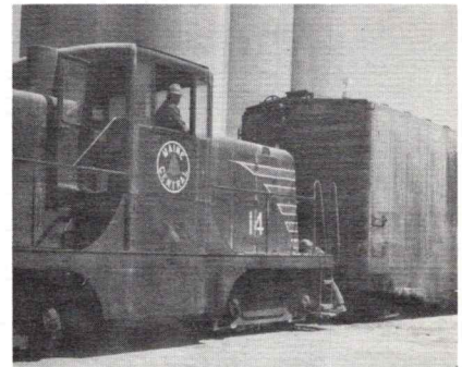
Maine Central Engine 14 leased to the Martin Marietta Cement plant shown shoving cars into the silo for loading. Cement plant used this unit while their remote radio controlled locomotive was being overhauled.
