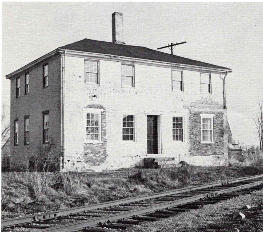
Renovation underway to restore the building to its original appearance. 1974 saw the bay window removed and door returned to its original position in center of the building.
