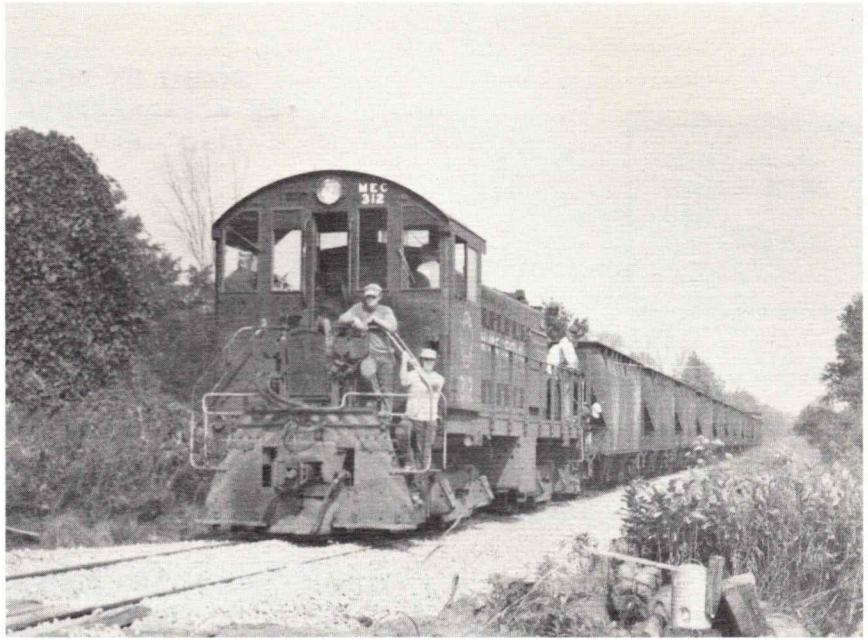
This was the first train that went to Scott Paper Company's new plant area at Hinckley. The crew is putting new ballast on the roadbed.
